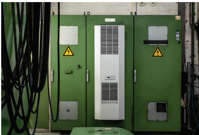
Picture above: Cooling unit DTS 6X1E on the control cabinet of a milling machine.
