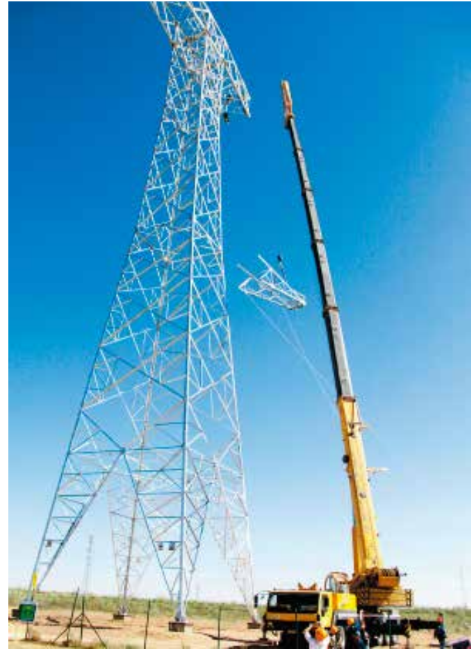
UHVDC line under construction
