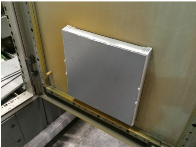
The filter fans from Pfannenber are fully sealed so that no air can enter them.
