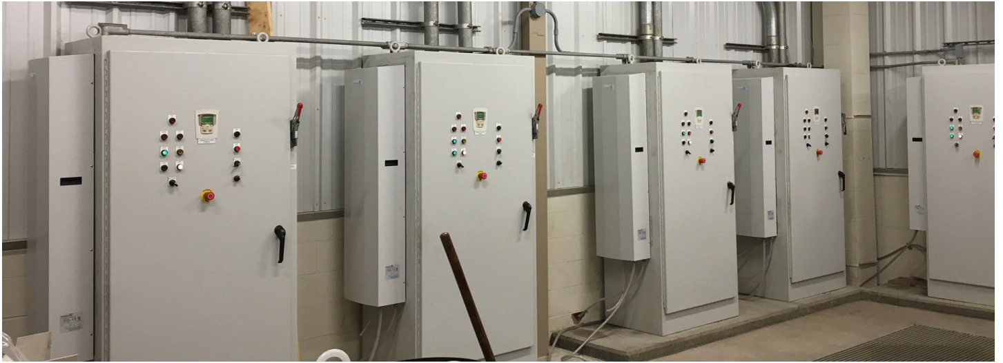
Pfannenberg air-to-water heat exchangers in the pump control room of a wastewater treatment plant.
