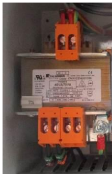
Picture 6 - Unit CE: Factory setting 400/3/50
